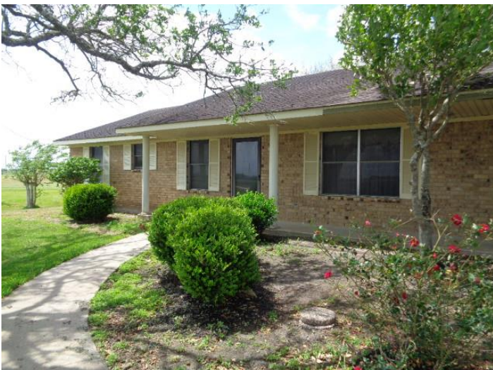
Front door, porch & front sidewalk
