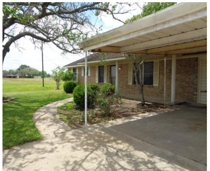
Attached carport/concrete driveway & front sidewalk
