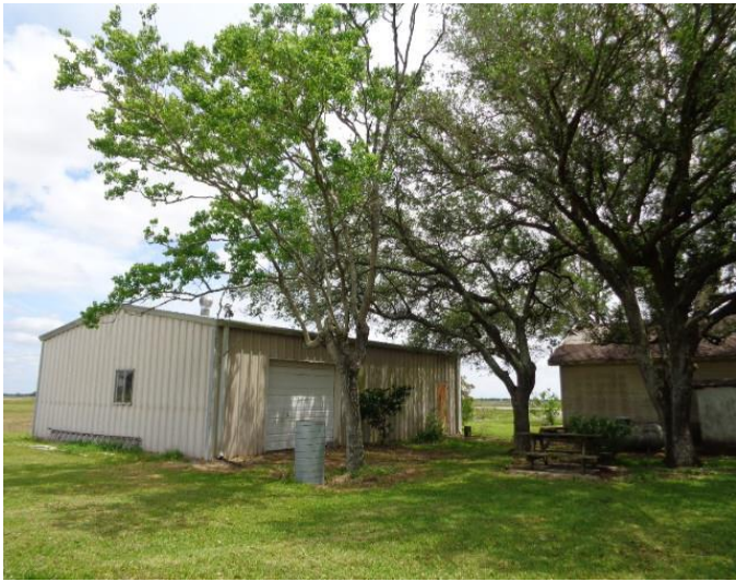
View of metal building from backyard
