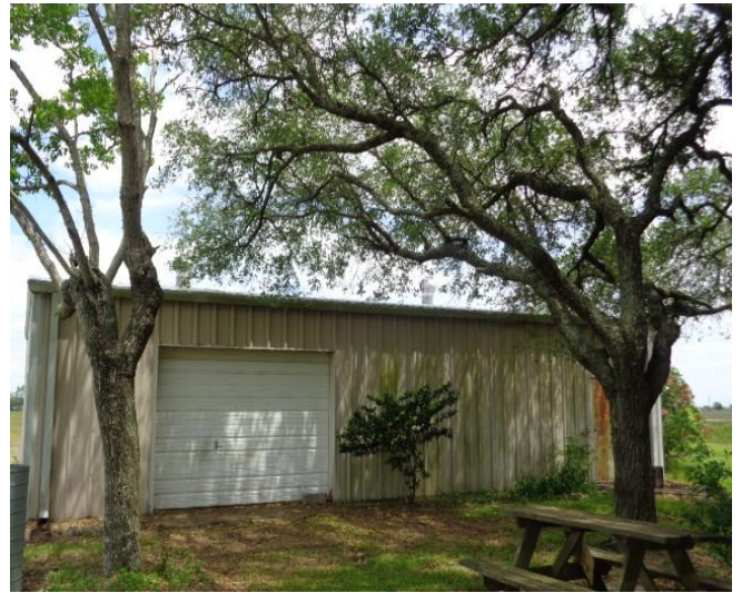
Overhead door on side of metal building
